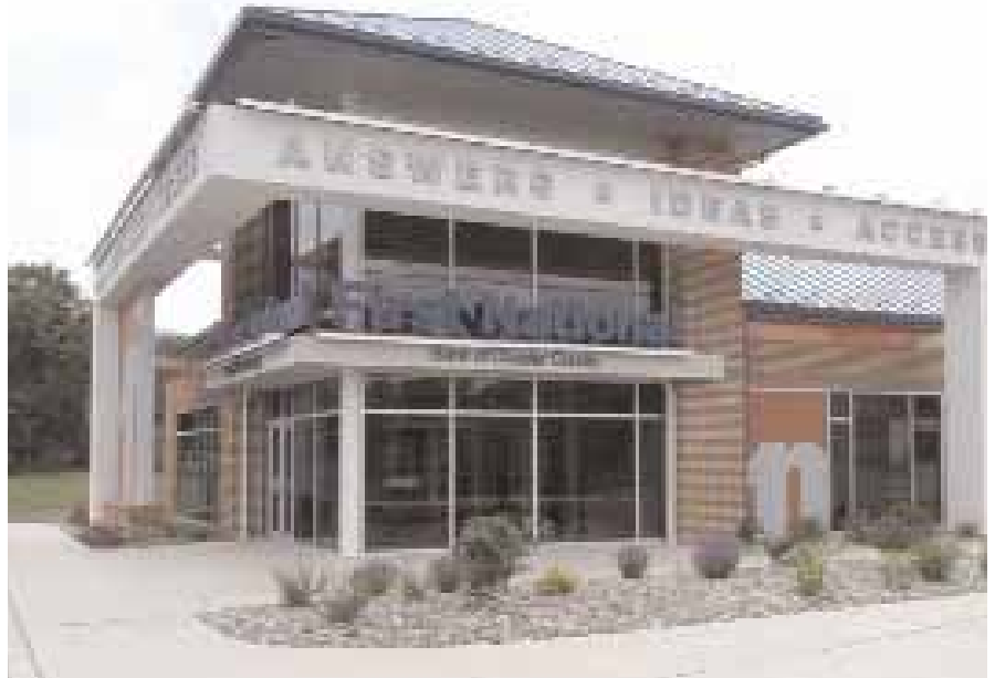
The brand—and retail experience—work from the outside in at this branch of First National Bank, West Chester, Pa. The “answers, ideas, access” message informs the design of the interior, picking up similar messaging and color themes.
